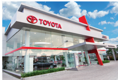
AUTO 2000 ELECTRICAL INSTALLATION
